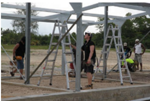
Students at work on the frame construction
